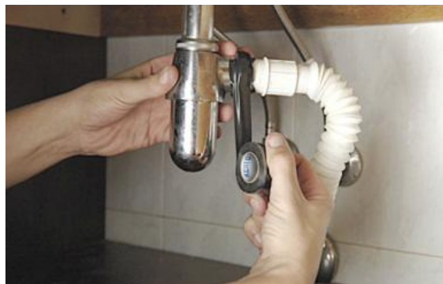
Reparation af revnet plastic studs
